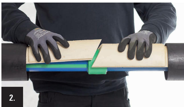
2. Assembly of the PUR-insulation shells: Push one of the PUR insulation shells marked 1 and 2 mutually in the cavity of the casing pipe, join together and turn to the underside.
