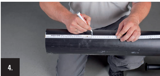
4. Mark the skinning length of 22.5 cm from the pipe end on the casing pipe.
