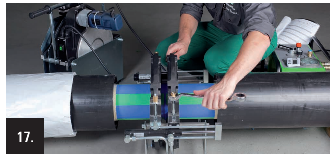
17. After the end of the cooling period the pressure is released at the hydraulic system. Then the mounting clamps are disconnected and the clamping device is removed.
