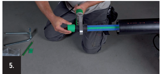
After the heating time pull off the welding socket and the pipe end from the welding tools.
