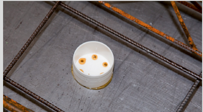
Base part of sprinkler outlet Art. no. 3090000005 for concealed sprinklers. Attachment with hot-melt adhesive.
