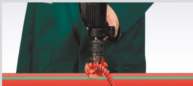
Drilling through the pipe wall
