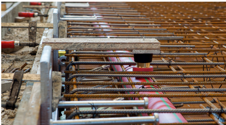
Prefabrication concrete wall
