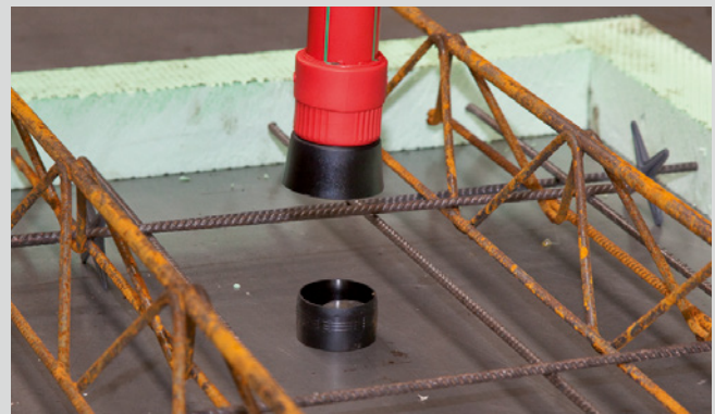
The upper part of the sprinkler outlet with pipe connection is attached to the base part of the sprinkler outlet.
