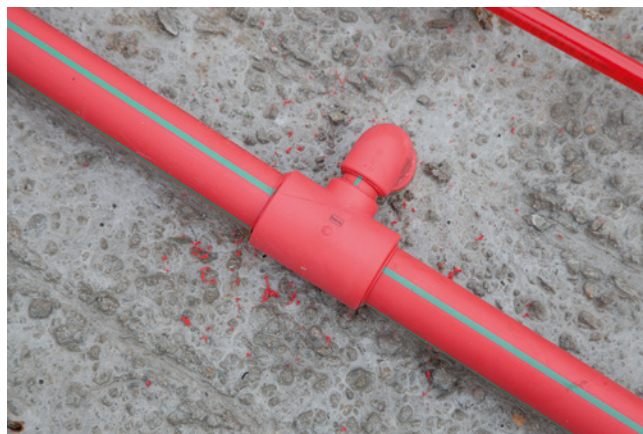
Assembly precast concrete ceiling
