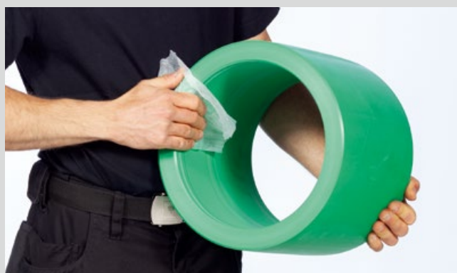
Clean the electrofusion socket's inner surface with a lint-free cloth or paper. Remove moisture that may occur immediately before the welding process again.
