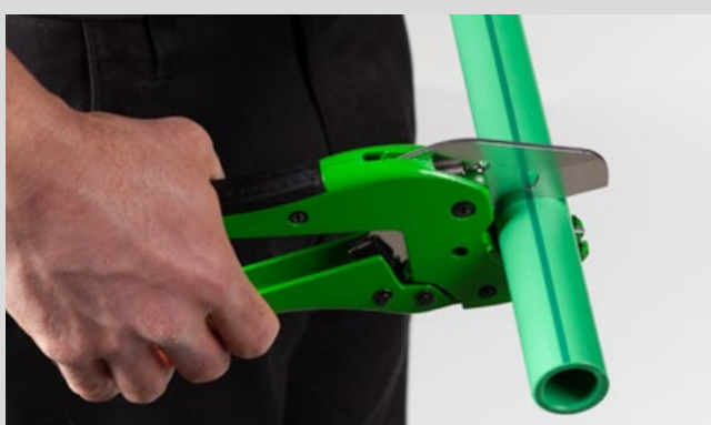
Cutting of the pipe
