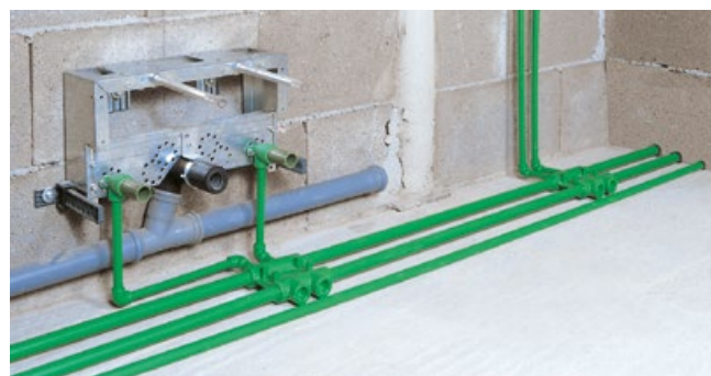
Floor distribution with distribution blocks
